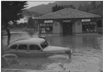
Downtown San Anselmo (Bollinas Avenue) during the 1944 Flood
