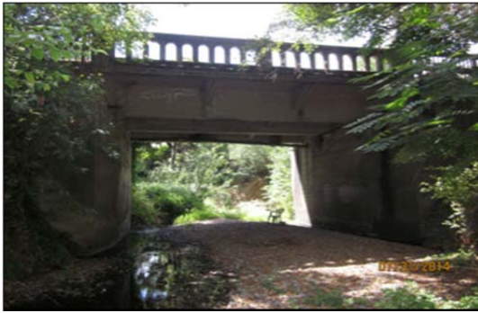
Madrone Avenue Bridge
