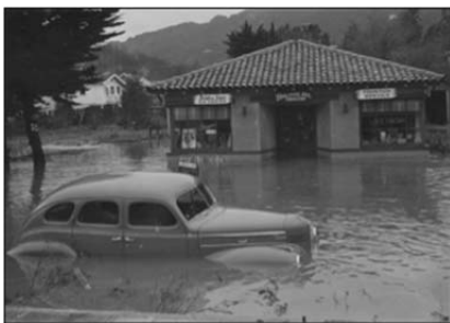
Downtown San Anselmo (Bolinas Avenue) during the 1944 Flood
